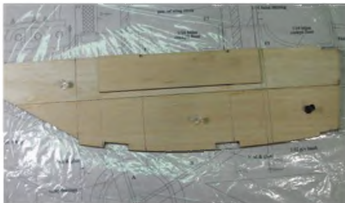
The sheet side parts joined and the c/s strut doubler glued in place. This enables you to fit the c/s struts after the basic fuselage is complete.
