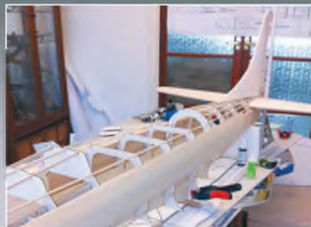
Fin and tail fixed to the fuselage and sheeting commenced.
