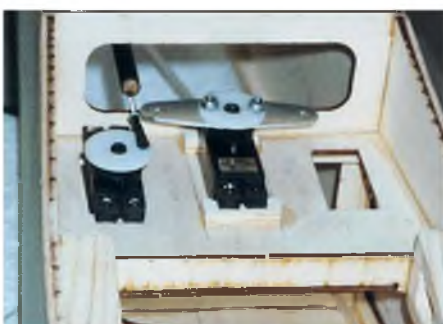
Fitting the control cables and elevator rod - before fitting the cross bracing.
