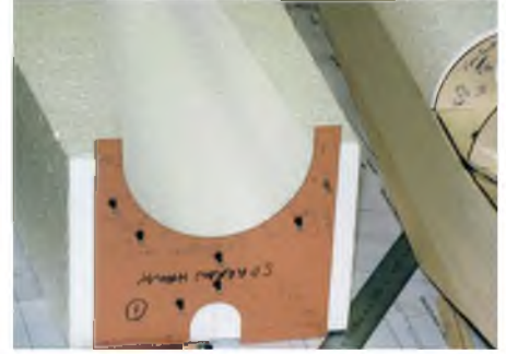
Cutting and fitting the foam decking.
