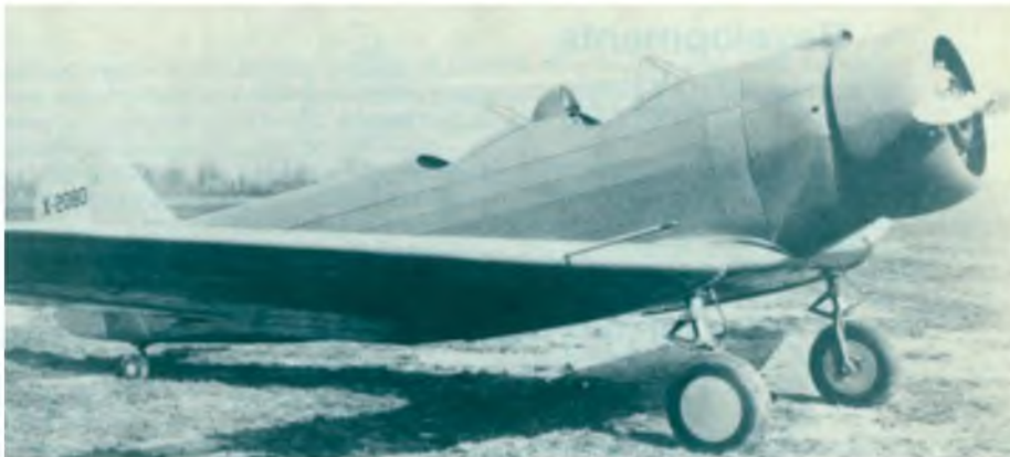
Where it all began, the prototype NA-16 as it first appeared, with open cockpits. The fixed undercarriage had no leg fairing and wheel spats.
