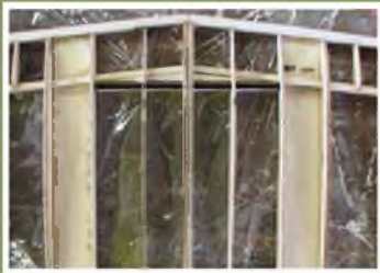
A clear view of how the wedges and braces work once the wing panels are joined.
