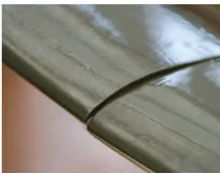
One of the outer top wing panel mismatch with the centre section at the leading edge.
