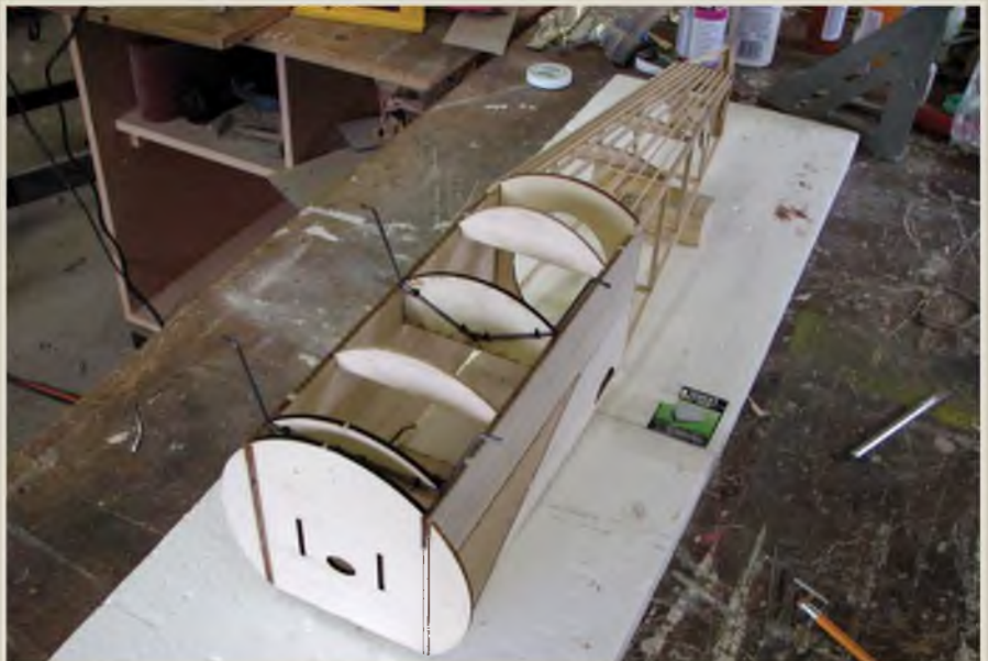
Can you spot the 'deliberate' mistake? Yes, those c/s struts are in the wrong positions. At least it shows how they're bound in place.
