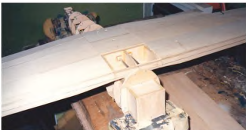
Mating the wing to the fuselage to drill the retaining dowel and bolt holes.
