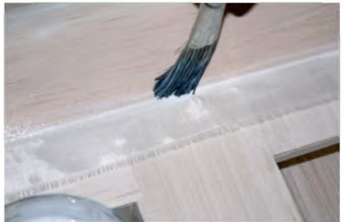
At sharp changes in contour, work the cloth into the corner with the tip of the brush.
