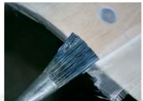
Finish off by using a loaded brush to smooth down the overlap 'flaps' to a smooth surface.
