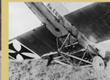
The fragility of WWI aircraft is well illustrated by this unhappy E.III which has nosed over. But such damage could be easily rectified by skilled riggers.
