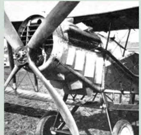
After WW1, the use of the Bristol F2B overseas in countries including India and the Middle East, led to cooling problems in climates well in excess of those encountered on the Western Front in Europe. One cure investigated was the application of extensive cooling louvers around the engine cowl.
