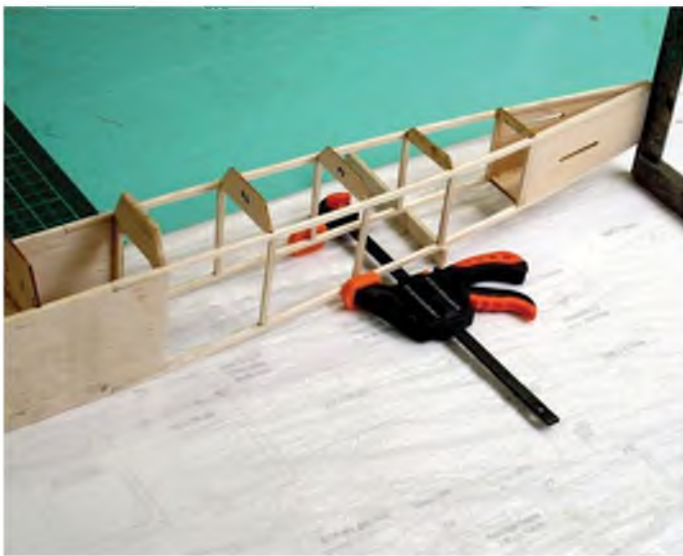
Aligned over the plan and with the tail packed up the tail is pulled in and the rear formers fitted.
