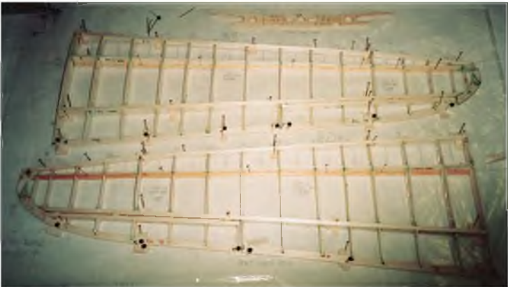
Upper wings under construction.
