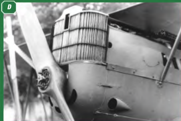
showing the radiator, cowling and engine installation of the example held on display at the Australian War Memorial Museum, Canberra
