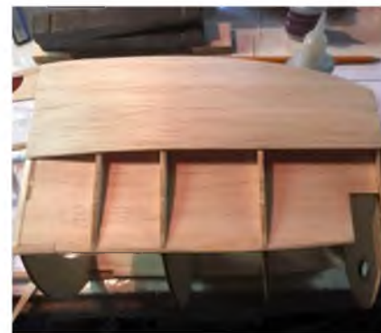
By comparison, the sheeting going onto the side with the slight 'hump'.
