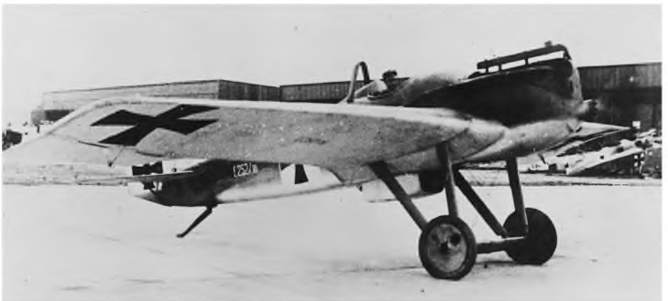
The most photographed of the group, E252/16 warms up on the hard standing at Adlershof. Performance was improved somewhat by the installation of a 160 hp Mercedes D.III engine. Only the second J2, E252/16, was fitted with a machine gun.
