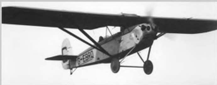
Widgeon III G-EBRQ was registered in July 1927 and was fitted with a five cylinder Armstrong Siddeley Genet radial engine. During 1928-29 owner Sqn Ldr 'Daddy' Probyn made a 4,200 mile tour, taking in Pisa, Tunis, Oran, Madrid and Biarritz. 'RQ' was withdrawn from use at Hinaldi, Iraq in January 1936.
