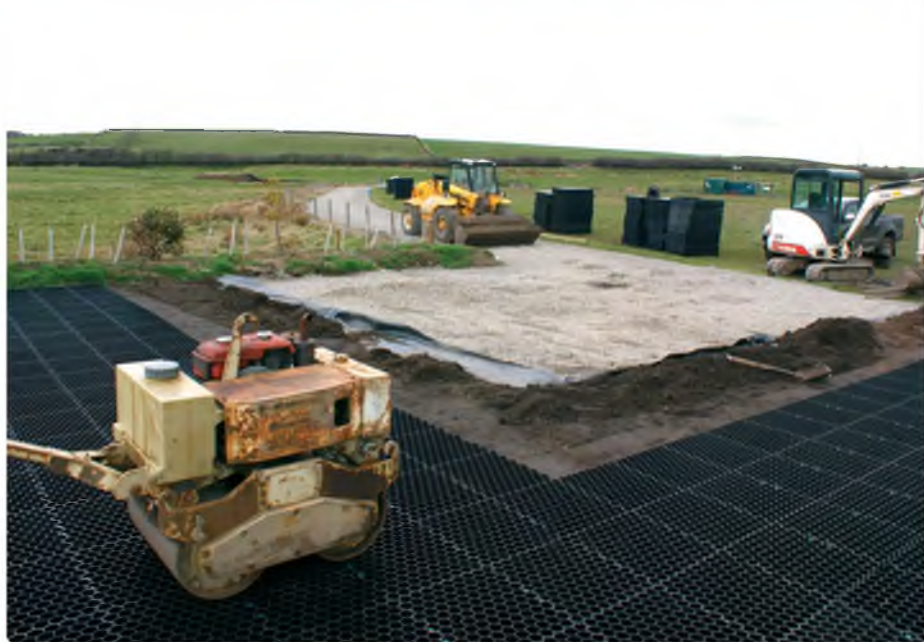
New track to car park, with the pit in the old position
