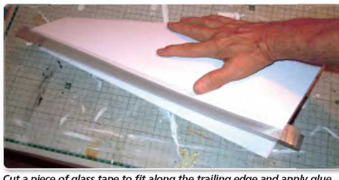
Cut a piece of glass tape to fit along the trailing edge and apply glue to the top of the spar and the T.E. chamfer
