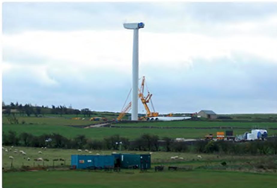
Turbine under construction
