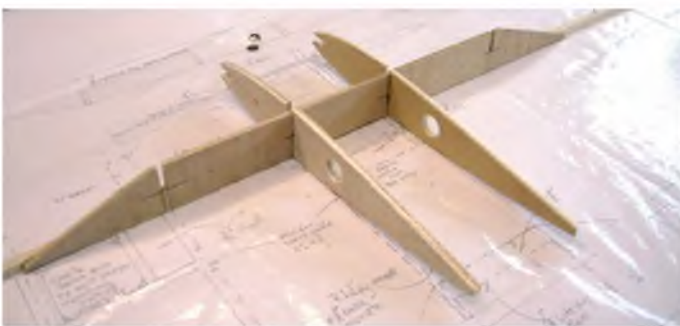
Start building the wing upside down at the centre section
