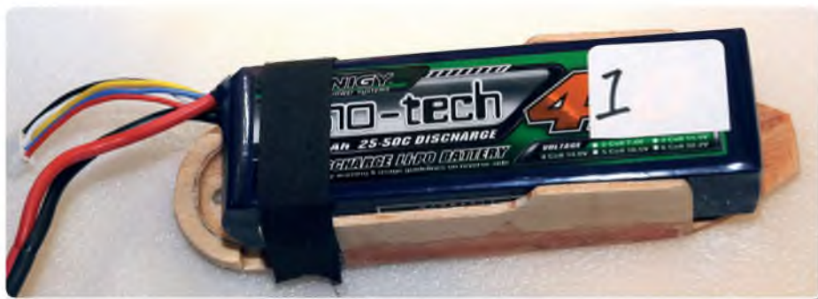
A new, slightly larger battery in place with strap
