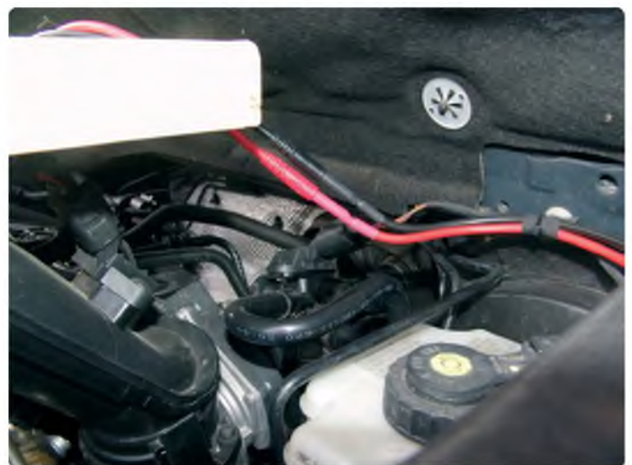
Supported by a plastic body clip, the wire leads with their heat shrunk jacks are running towards the board
