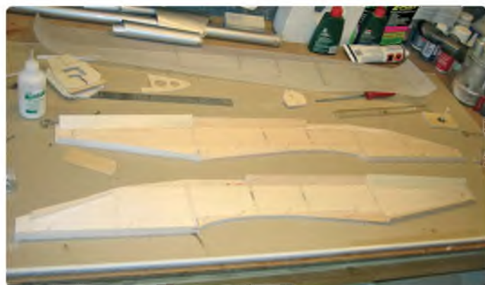
Fuselage side assembly with triangular sections, 3/16" wing root doublers and 1/4" front nose doublers
