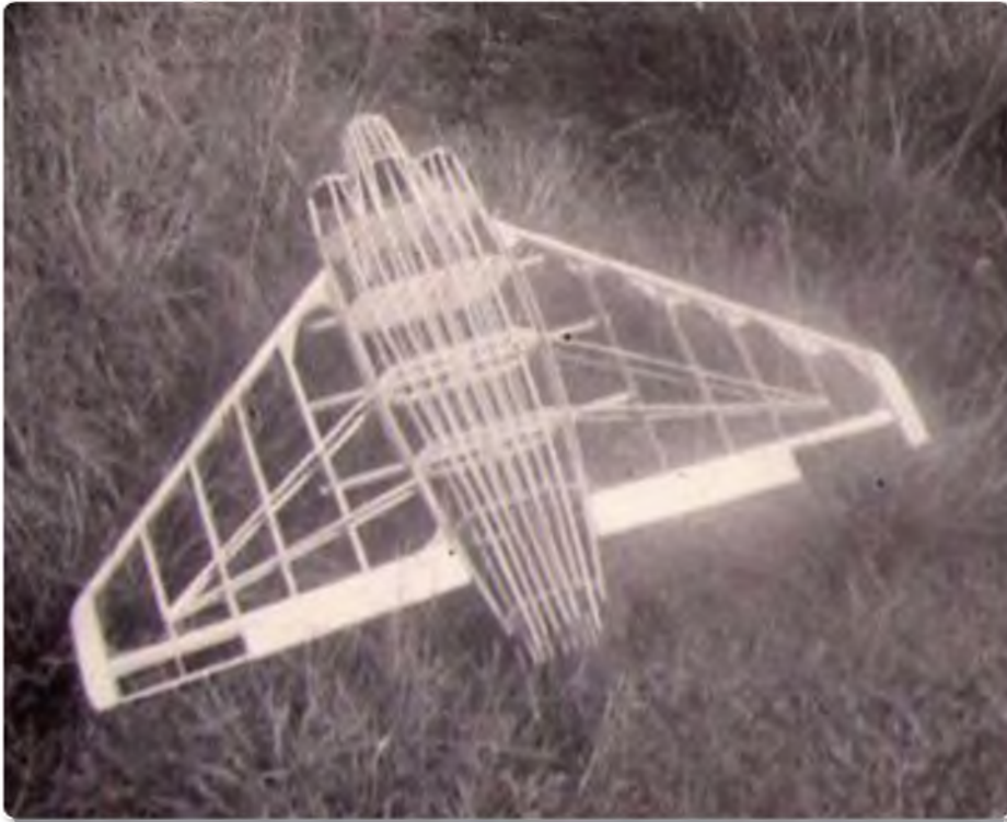
Jet models were popular. This photo is (I think) of a Keil Kraft Gloster Javelin prior to covering
