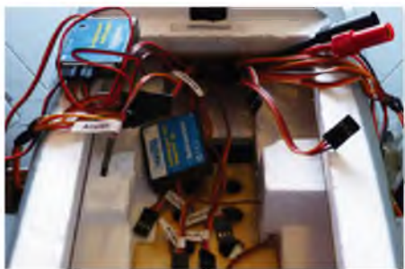
There are a lot of extension leads to connect. Use of a 10-channel receiver reduced the need for 'Y' leads
