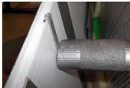
Slotted across the side flutes, the hangers also afford some more anti-squash resistance
