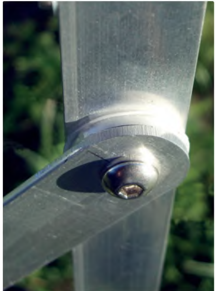
One end of each two-part cross brace needs a spacing washer
