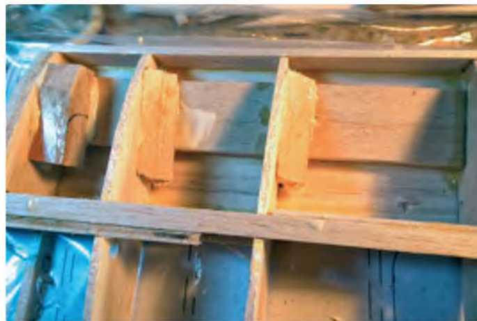
Beech block and triangular stock glued in place
