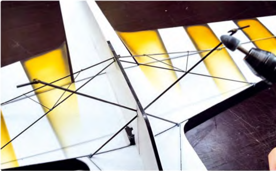
For the axles use 1.5 mm thick carbon rod. Mount light wheels as shown. Place the model on a flat surface and once everything is straight and level cut the axle and trim any sharp edges with a precision drill/grinder as shown
