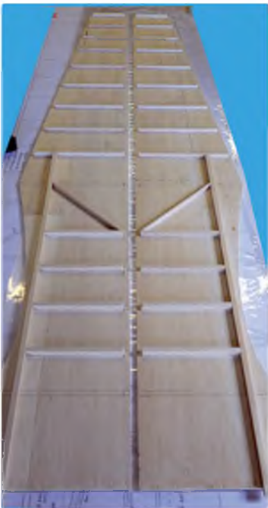
Completed side frames with uprights and stringers added
