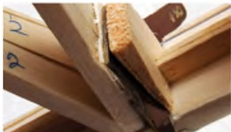
Paxolin horn epoxied between two wedges and glued into place
