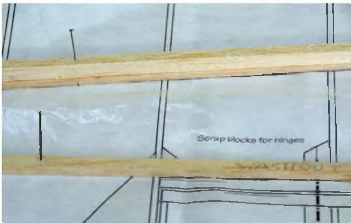
Pin the lower spar to the washout jig. They are separated by plastic sheeting to make sure nothing sticks
