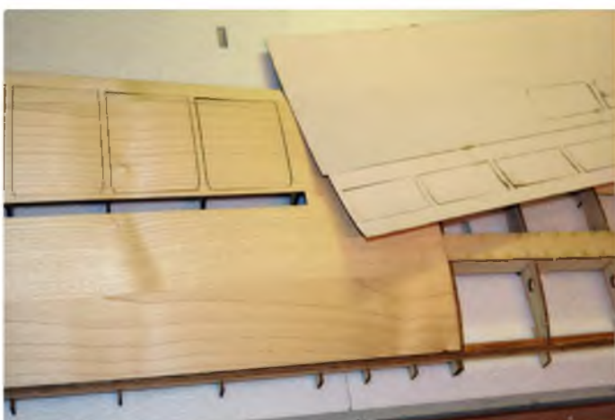
The wing is sheeted using pre-cut fabric backed veneer sheets, which provide a lightweight, strong and flexible surface. Note the upper ply capping strip applied to the vertical spars, which builds up into a very strong box section
