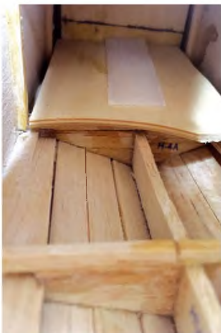
A floor for the battery, and the former at the front of it, were put in during the early stages of fuselage construction
