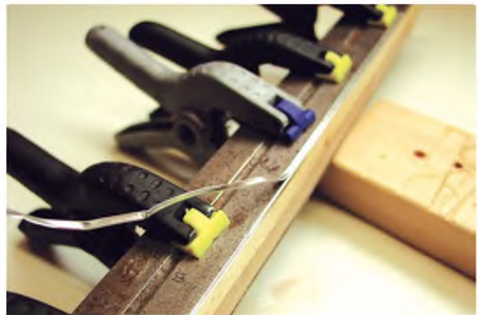
Making cockpit coaming. First clamp the material to a steel rule
