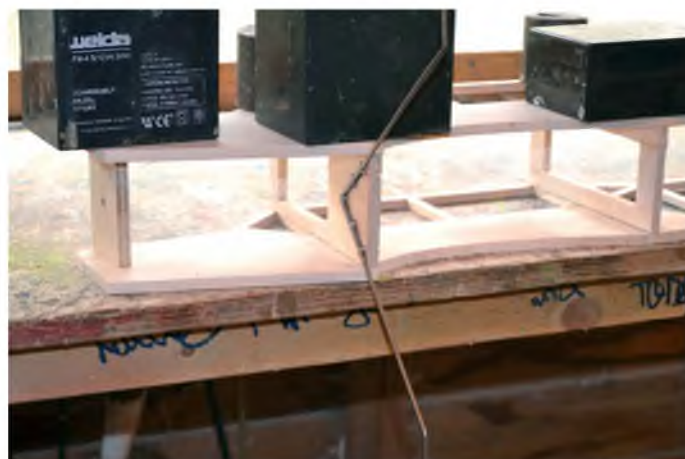
Weigh the fuselage down until the glue dries
