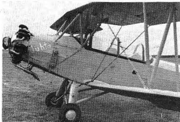
Covered cockpits on OH-VIJ at Kauhava, Finland, pale cream overall with white name on cowling. The canopy slides in one piece along special spine forming a dorsal fin. Right, is Swedish SK 12 serial 615 in 1940 regulation markings.
