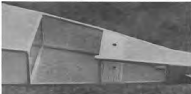
First job in rejoining that longeron is to tidy up the damage ready to accept a new piece of stringer.
