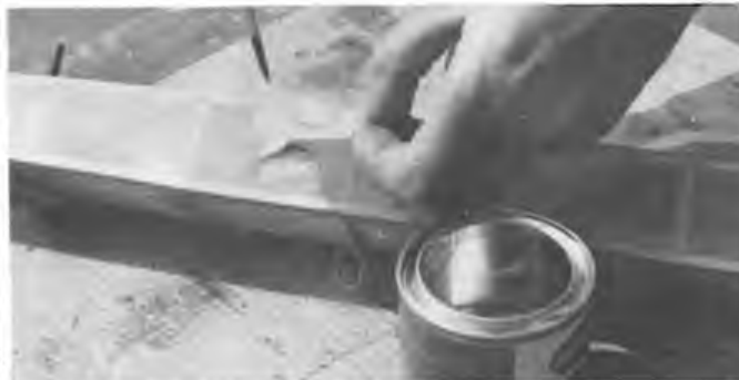
For small tears in the tissue, like this one, the panel need not be completely removed - a tissue patch can be doped over to secure the surface.
