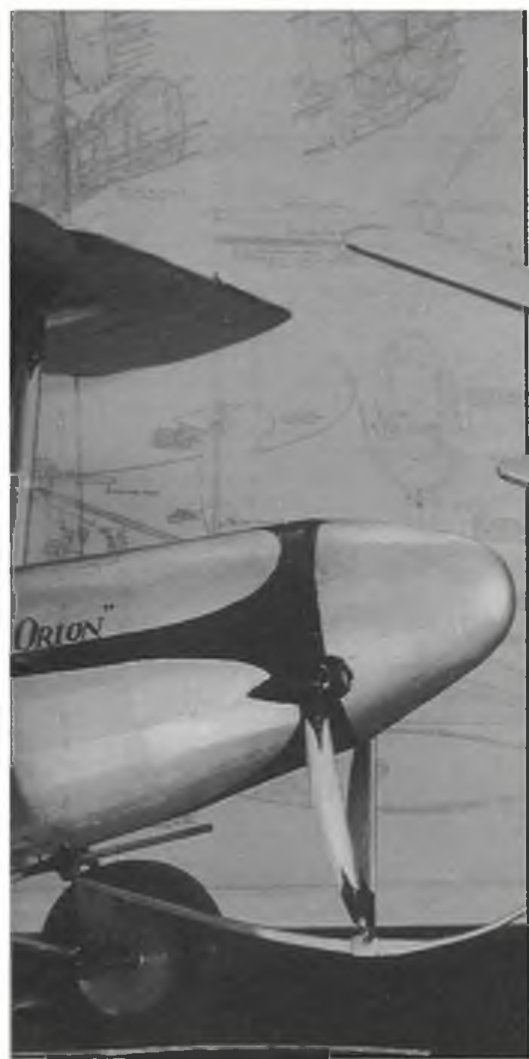
Above: Neat engine nacelle and fairing are evident. Covering has been stripped from port upper wing.
