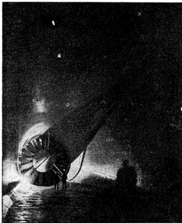
(Above.) Gargantua I Looking down the long return section of the Boeing Aircraft Corporation's wind tunnel. Below is a view of one set of "turning" veins. These veins, of airfoil shape, are hollow and filled with water to cool the airflow, which becomes hot at the high speeds at which the tunnel operates.
