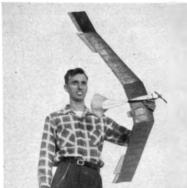
M. M. Gates's American contemporary, Donald C. Broggini, who has been writing a series of articles on Tailless Design in "Model Airplane News" is shown at left with the dethermaliser parachute extended from the centre section of his twelfth design. Readers will note that this model incorporates a cathedral centre section for down thrust effect, and also to raise the centre of gravity. The upraised and cambered tips aid stability. Above: Broggini's seventeenth and most successful design, with three of the trophies it has collected. It weighs six ounces, is 54 ins. span and has a .8 c.c. glowplug motor. At the Nassau Plymouth Eliminations it amassed a three-flight total of 12 mins. 24 secs in the half-A open contest.
