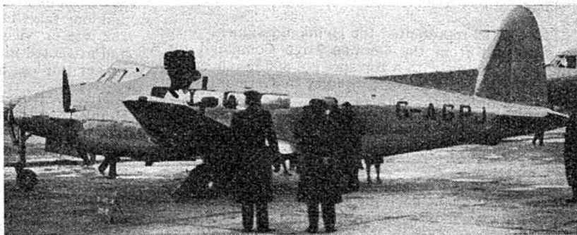
(Above.) Second Thoughts. When on view at Radlett last February, the prototype D.H. 104 Dove was seen to have a revised and extended fin fillet.
