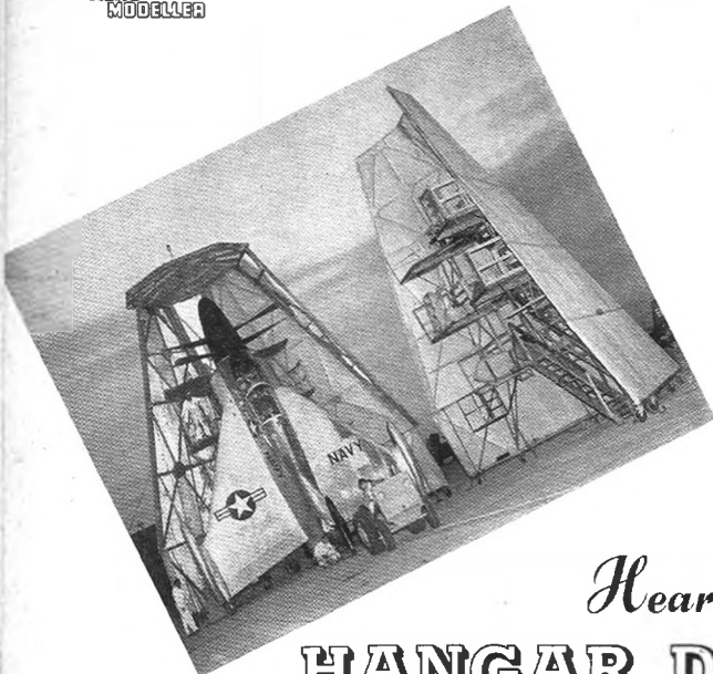
New style in Hangars is the isosceles-shaped "clam - shell" with triple decked working platforms for the Cameroise XPV-1 "Pogo." Hangar rolls on wheels so that it can be taken to the aeroplane if needed.
