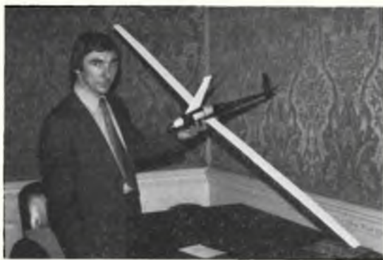
Peter Wright of Melton Mowbray is completing his second MP aircraft which, like his first, employs carbon fibre-reinforced epoxy extensively. In fact, the 'Micron' is almost all plastic and has been produced in moulds so that others can be made later. Aspect ratio is 'over 40:1', and the vee-tail has butterfly rudder-ventrator controls. The 'Micron' will have a 9ft. diameter propeller and what promises to be high efficiency performance from the narrowest wing yet seen on a man-powered aircraft. The whole design and construction has been a solo effort and included making the scale test model which Peter is seen holding at the Royal Aeronautical Society Symposium.
