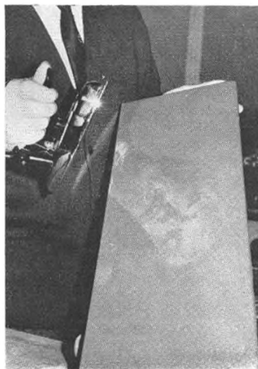
Using domestic iron set at "wool", heat seal all wraps with gentle rolling action, start at centre, working to ends.
