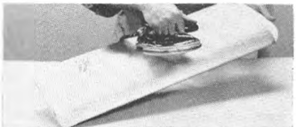
3. Glide iron over surface to pull up taut.
