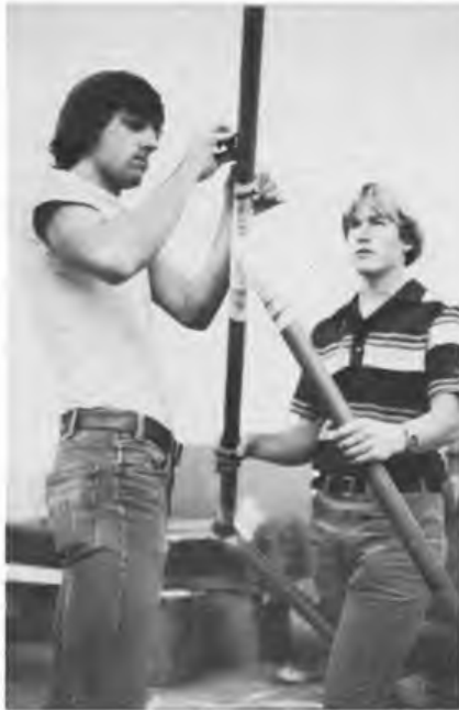
Left: hang glider flyer Carlos Miralles (left) and model flyer Bobby Curtin, assemble fuselage frame tubes; junctions are well reinforced with extra Kevlar cloth and epoxy. Below: Blaine Rawdon, member of Cross-Channel Albatross crew, was responsible for most of the structural design on Solar Challenger, seen here on the tube wrapping machine strapping with Tedlar.
