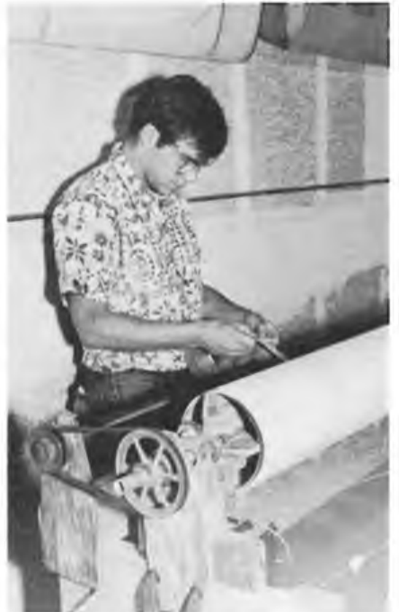
Left: hang glider flyer Carlos Miralles (left) and model flyer Bobby Curtin, assemble fuselage frame tubes; junctions are well reinforced with extra Kevlar cloth and epoxy. Below: Blaine Rawdon, member of Cross-Channel Albatross crew, was responsible for most of the structural design on Solar Challenger, seen here on the tube wrapping machine strapping with Tedlar.
