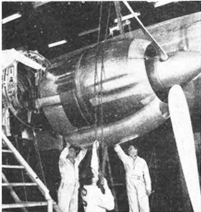
A Wright Duplex-Cyclone is installed in a Lockheed C-69 Constellation. A complete change of power-egg can be effected in 27½ minutes. (Lockheed photo.)
