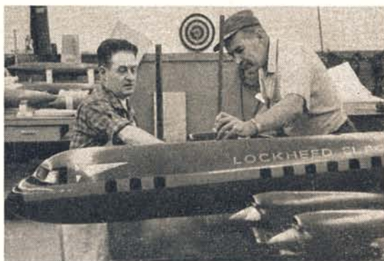
Back at work in Lockheeds on Tuesday after flying at Woburn on Sunday, Bob Palmer checks a mahogany wind tunnel model of the Electra which he spray painted in blue and grey.
