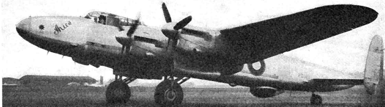
A. T. P. Photo. SHETLAND PROTOTYPE: The original military Shetland with the turrets faired over.
