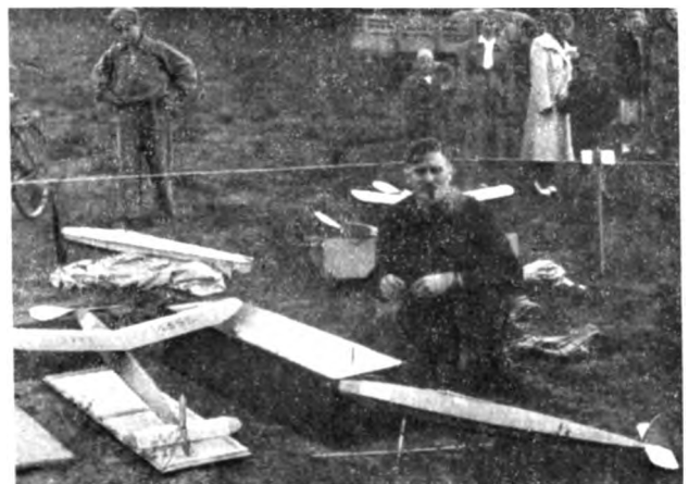
Below: The Belgian corner with Deschepper and pipe, in centre. Diamond fuselages, with unusual built-up 'spine' wing mounting platforms were features of the Belgian models. Deschepper used a variable pitch prop on his entry.
