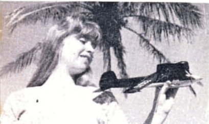
Left, Sandy Pinkert with Don Pinkert's 173 m.p.h. S.T. .29RV speed model, Florida. 60 per cent Nitro, 20 per cent Castor Oil, 5 per cent N. Benzine, 15 per cent Methanol. Below left, S.T. 40RV powered "Hoptee" by Art Adamisin, Detroit. Note long tank with Quick Fill Valve. Below, John Kilsdonk, "Hoptee" designer M.A.N. plan 67A.
