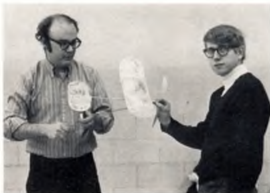
When winding, your assistant should hold the dual bearing, prop hub between finger and thumb, whilst you apply the turns from the rear using a geared winder.
