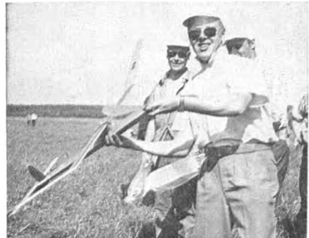
Russian influence evident on R. Holsaess' Wakefield at German Nats. Has full span turbulators taper sheet on L.E. and tubular fuselage, though not the outrigger prop blades used by Matvejev
