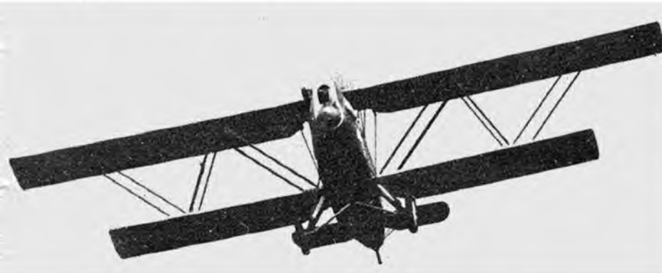
Early photographs of Parnall Elf show distinctive Warren girder wing bracing in head-on flying shot above. Full length top wing ailerons clearly visible at right, with full length hinge on lower wing to permit wings to swing back for storage. Left: fin and rudder hinge line differs from restored machine at Shuttleworth, "Air Portraits" & "Flight" photos.
