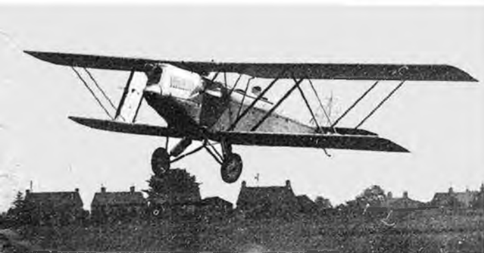
Early photographs of Parnall Elf show distinctive Warren girder wing bracing in head-on flying shot above. Full length top wing ailerons clearly visible at right, with full length hinge on lower wing to permit wings to swing back for storage. Left: fin and rudder hinge line differs from restored machine at Shuttleworth, "Air Portraits" & "Flight" photos.
