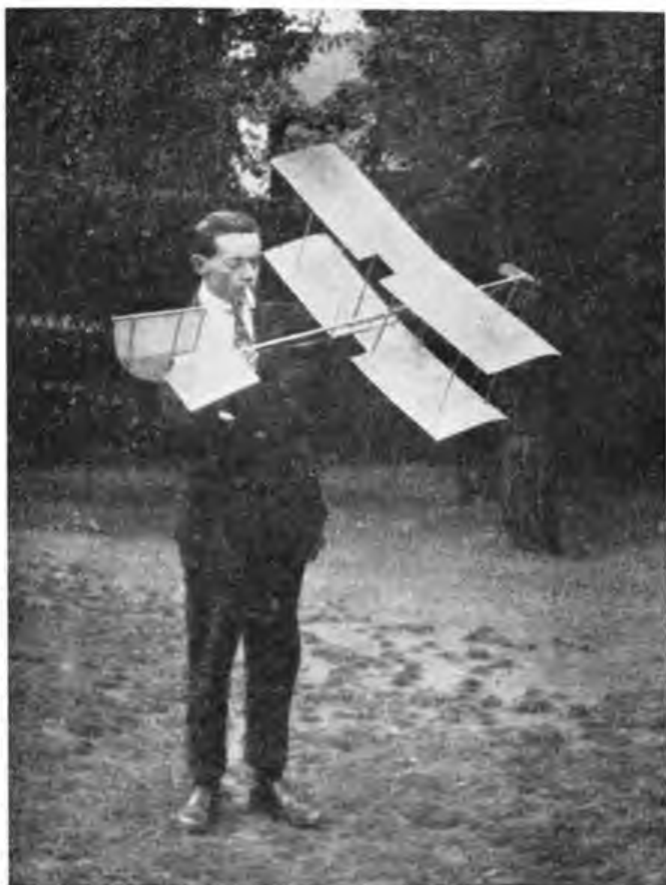
Here is picture 1, taken about 1915, and showing the Author holding one of his early machines. Construction would be mainly of birch or spruce. The wings, though cambered, were covered only on the upper surface. Straining wires of steel kept the main spar rigid.
