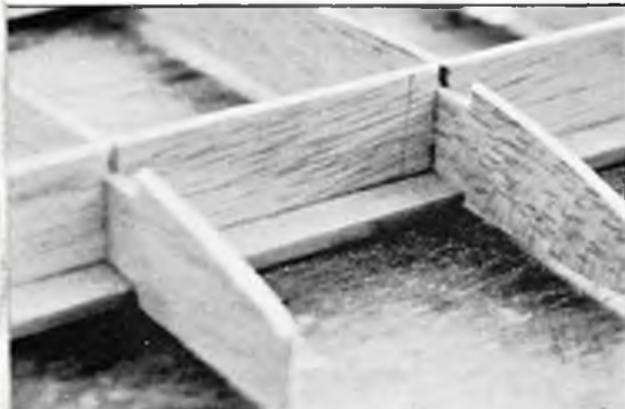
Full depth wing spar. The bottom spruce spar is glued to the vertical web before fitting the wing ribs.
