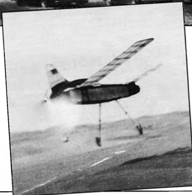
Above: Al Backstrom's 27in. rubber powered Arup. Designed by Gordon Englehart, this model was originally described in the September 1936 issue of Model Airplane News . Left: This pusher canard made by Mr. Hill of the Croydon and District MAC in 1937 is caught by the camera as it leaves on a 95.3 seconds flight. W. P H Goodsir, designer of the Frog Pterodactyl, belonged to the same club.
