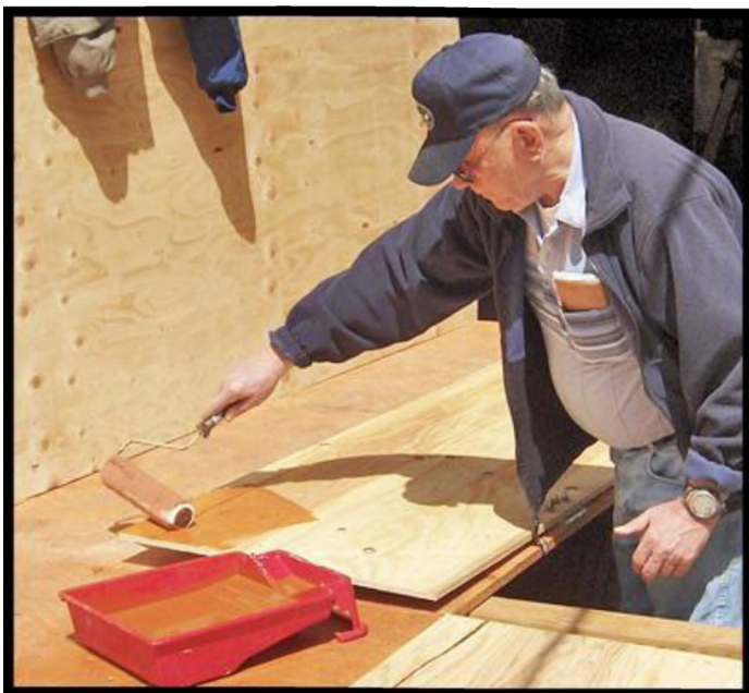
Chuck Kentfield Rolls On the Wood Preservative
