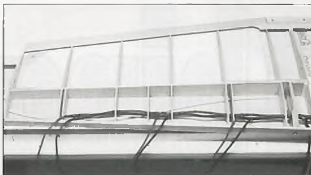
Wiring for motors is built into a conventional D box wing.
